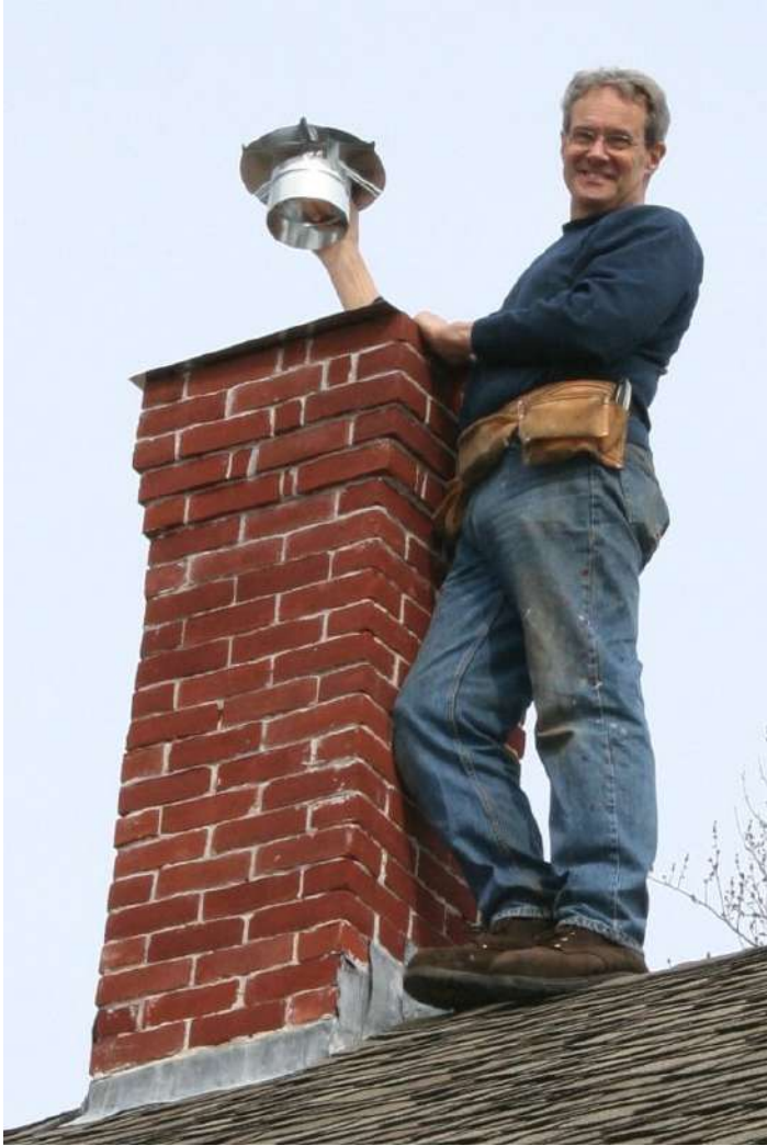
Warren Lampher working on the roof of Belknap School in 2009. Photo by Beth Hurd.
