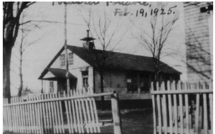
One of two "portable" schools in town, Pocasset School, pictured here in 1925, was a wood frame building resting on cinder block legs. At that time it served the children in the area centered on the Hartford Pike at Atwood Avenue. It is long gone. Photograph courtesy of Lora Clemence.
