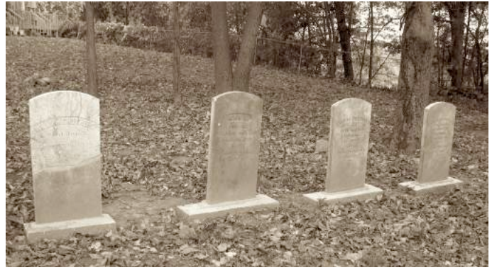
Some of the repaired and reset stones in Cemetery #60. Photo by Christopher Martin.
