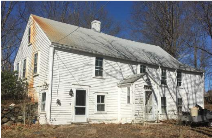
The south-facing facade of 218 Morgan Avenue. Photo by Christopher Martin.
